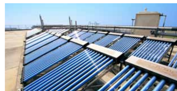
Solar water heaters installed on the roof of a hanger in HAECO 港機工程在機庫天台安裝太陽能熱水器
