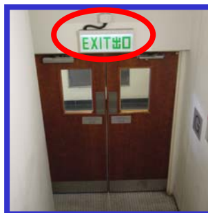
Staircase in BM
